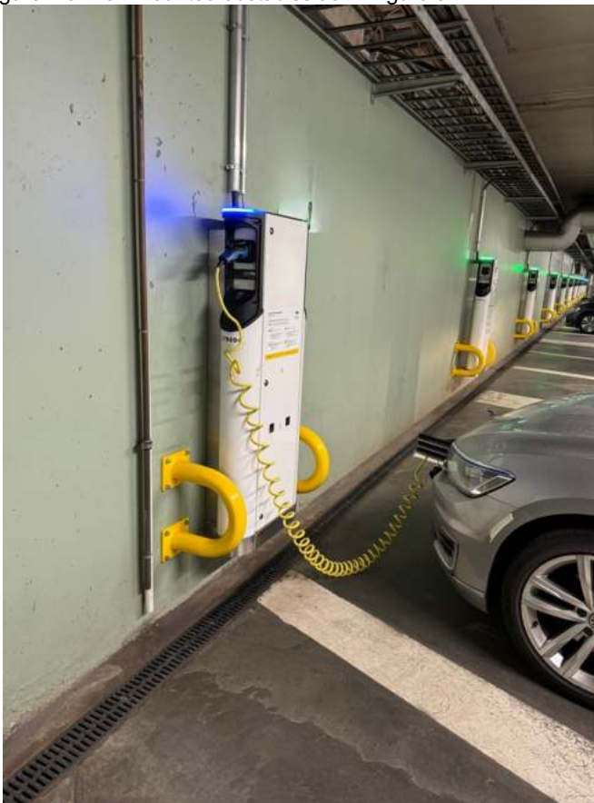
Fig. 5 Damaging the EV supply equipment by hitting them with the vehicle should be obstructed.
