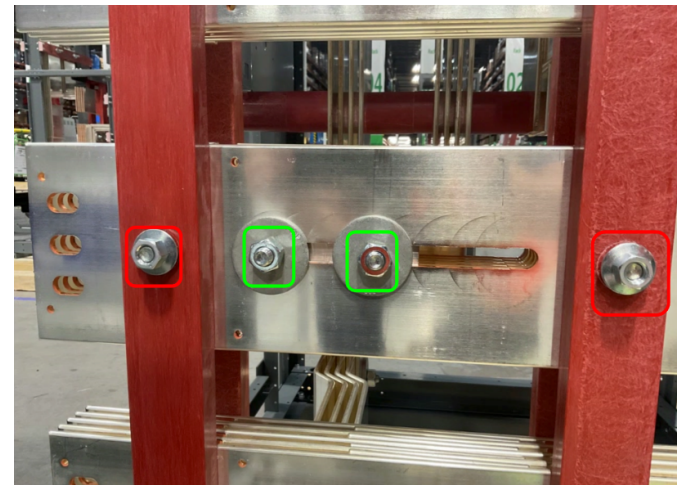
Fig. 15: Example of AI analyzed bolt torque. Green is approved and Red is identified as a defect.
