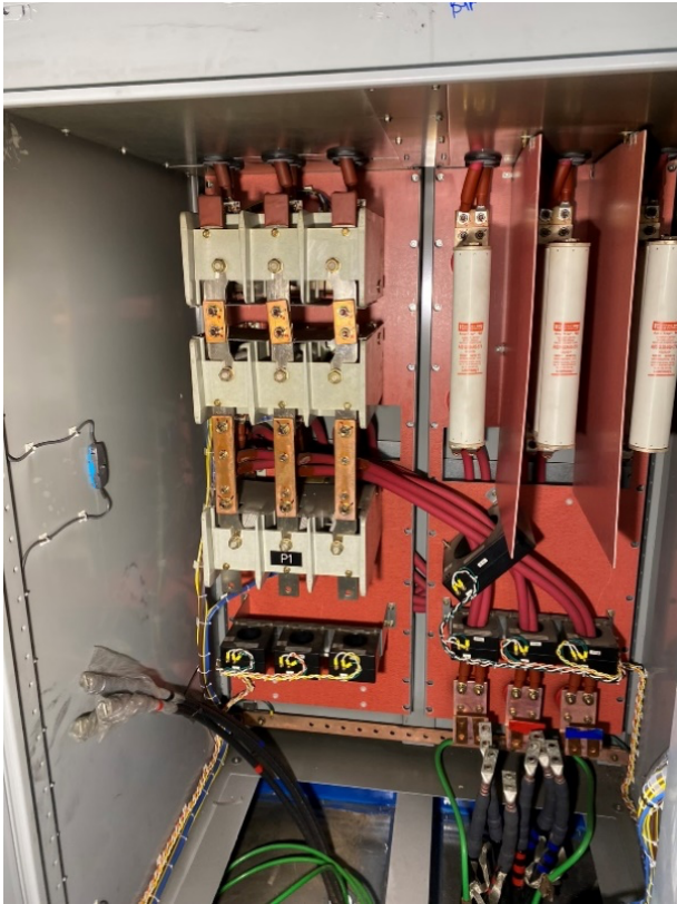
Fig. 2 Healthy Synch/Transfer Motor Starter during testing
