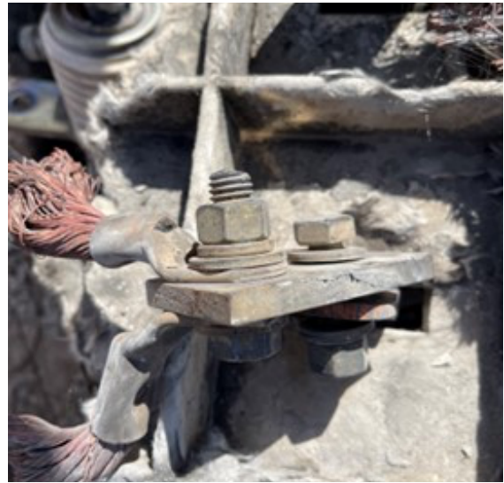
Fig. 3 Loosened "B" phase connection on the remnants of the bypass contactor
