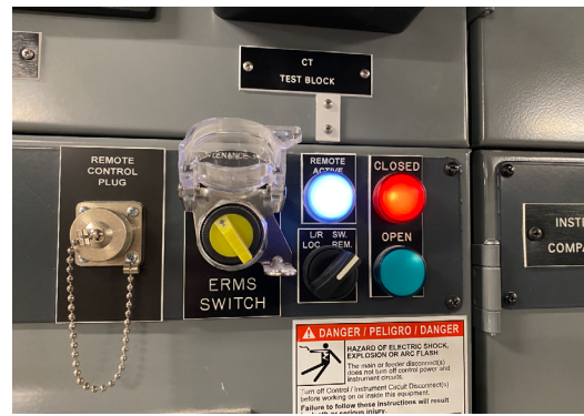
Picture 2 - The ERMS is the maintenance mode switch.
