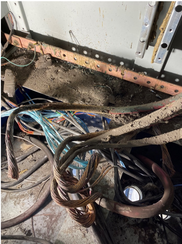
Fig. 5 Burned out enclosure
