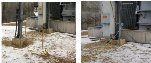
Figure 8 – Example of unsecured vs secured TPG jumpers
