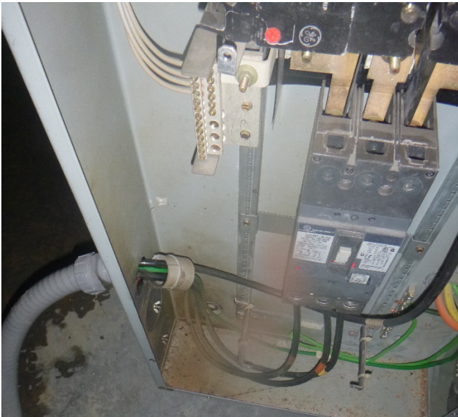
Fig. 3 Photograph of improper installation Used with consent of the Photograph Owner.
