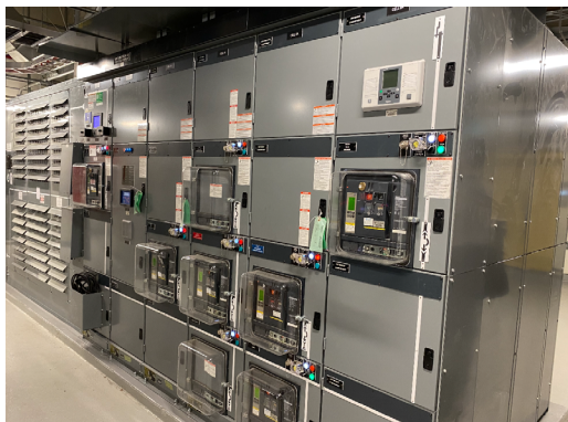
Picture 1 – Hospital Low Voltage Switchgear
