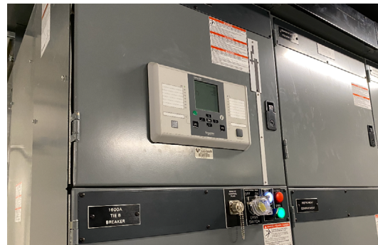
Picture 3 – Example Stand Alone Arc Flash Relay Installed
