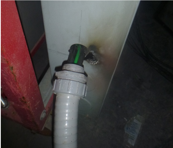
Fig. 2 Photograph of arc flash event Used with consent of the Photograph Owner.
