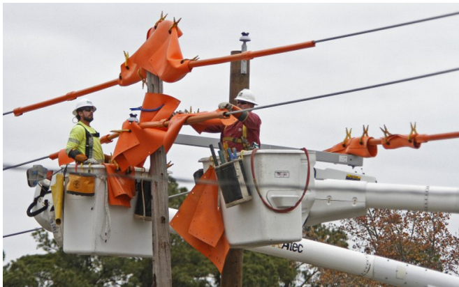
Fig. 4 – Linemen Covering Up Exposed Energized Parts
