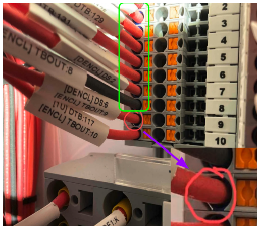
Fig. 13: Example of AI analyzed auxiliary terminations. Green is approved and Red is identified as a defect.
