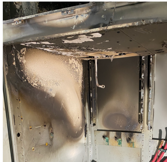
Fig. 4 Burned out enclosure
