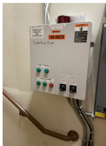
Figure 8: Retrofitted Mi-40 Duplex Controller
