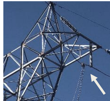
Figure 5 – Example of placement of multiple TPG jumpers on a single-phase conductor
