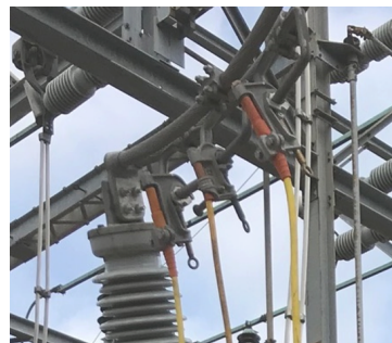
Figure 6 – Example of placement of multiple TPG jumpers on a two-bundled phase conductor
