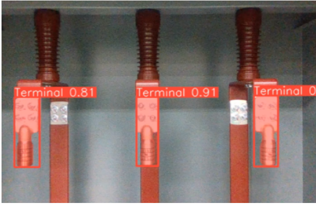
Fig. 2 Result of terminal instance segmentation in real time
